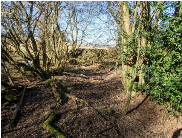
Figure 11: Wall at end of feature
