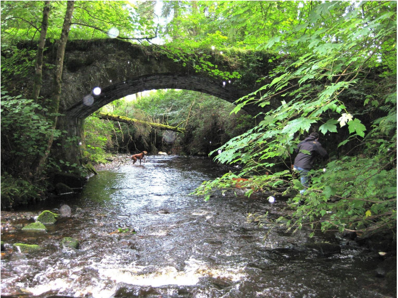
Fig. 8: Old Stone Arch Bridge Across the Nethan Water (2013, D.B. McCowan)
