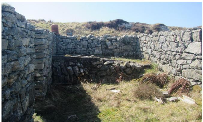
IMG\_1154 The interior of the house, looking south, showing the draining platform of the sheep dip. The dip tank was against the west wall (right) but has since collaposed, probably from frost damage.
